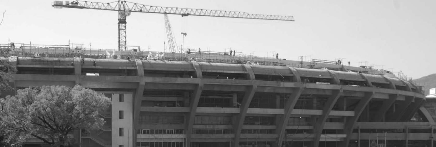
Maracanã renovations under way (Photo: Renato Cosentino)
